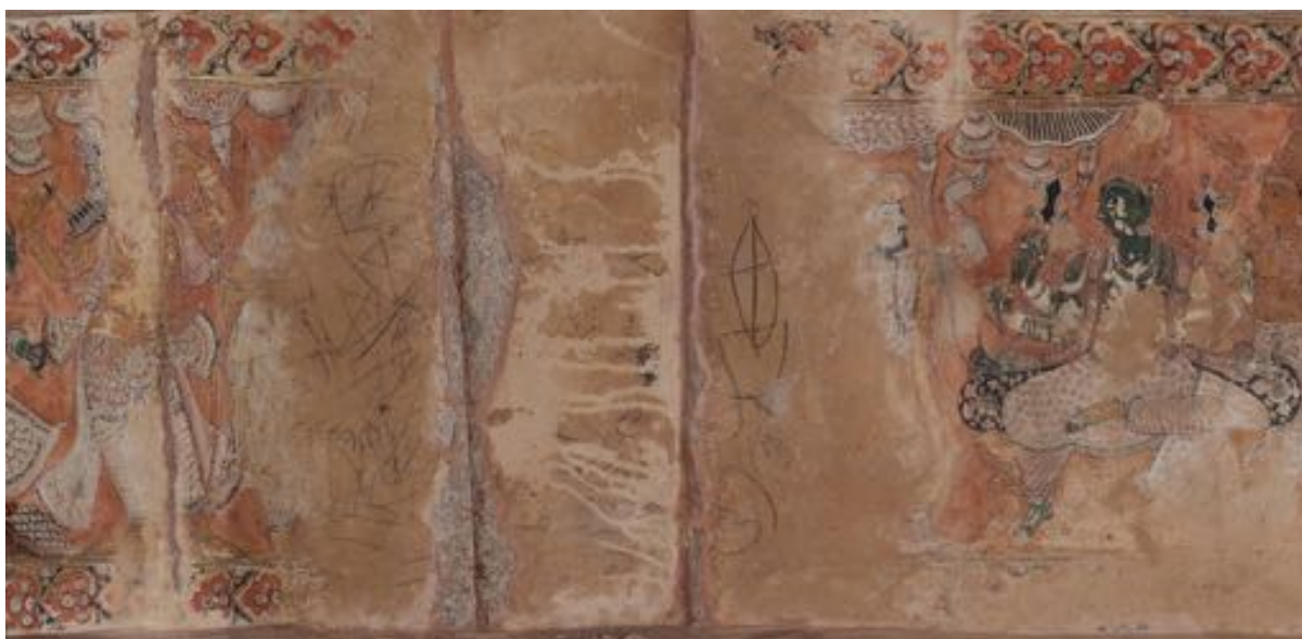
Figure 3: Damage due to Water Seepage and Vandalism; Veerabhadraswamy temple, Lepakshi Source – Vijayashree C S
